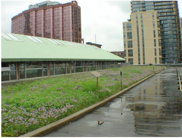
Figure 6.6 Semi-intensive Green Roof Example
