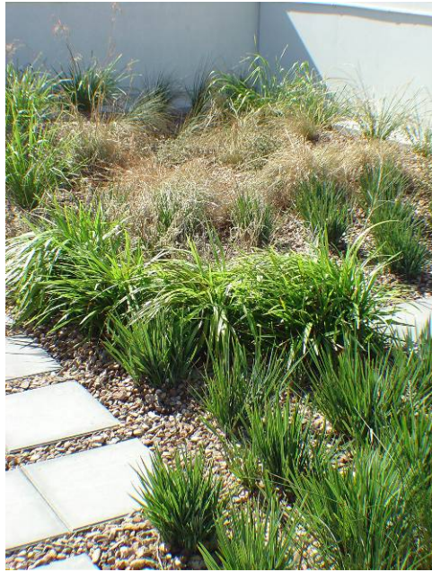
Figure 6.8 Intensive Green Roof, Hocking Place, Adelaide
